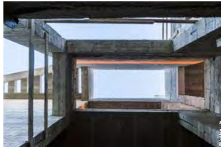
↑ Looking up the lightwell and solar chimney of the zero-energy family dwelling by Studjurban
